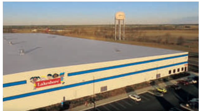
Our eastern distribution center in Midway, Kentucky.
